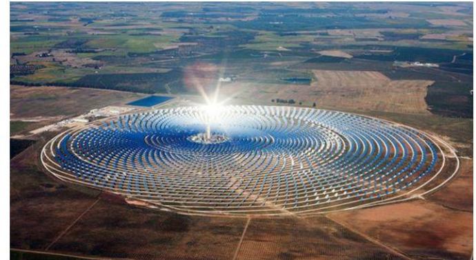
Fig. Solar Power Plant (Central Tower Receiver type) Up to 2000 °C
